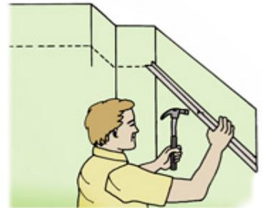
FIG. 6 - Use a level to apply the wall angle at a proper height around the room.
